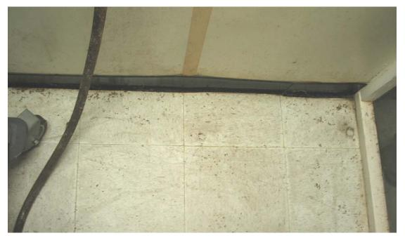
**Figure 1.2.7.** The mildew and mold growth on the walls and the floor of this insectary can stress mosquitoes causing them to be more susceptible to infections and less able to respond to changing conditions.
