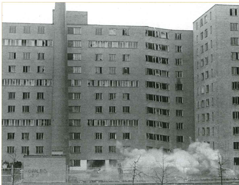
Demolition of the Pruitt-Igoe housing complex, March 16, 1972. Courtesy of the St. Louis Mercantile Library.
