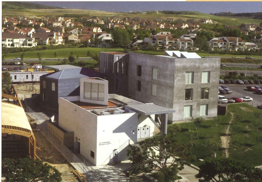
Information and Computer Science and Engineering Research Facility, 1989.
