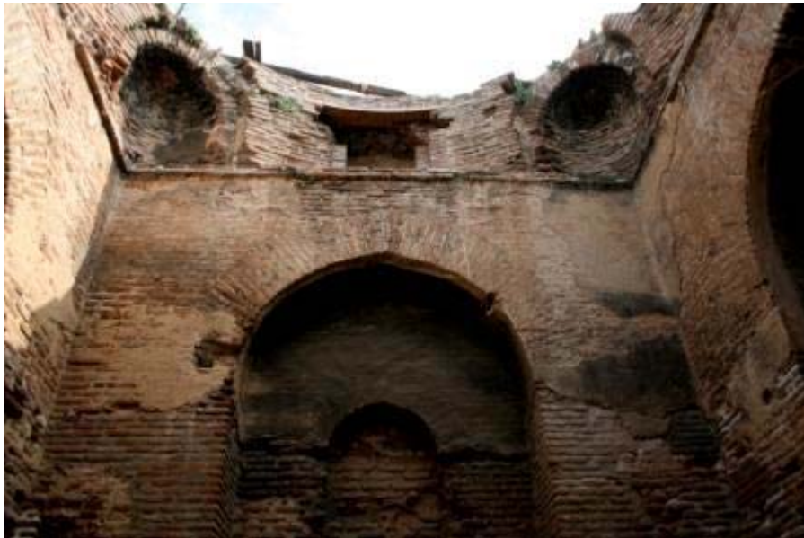
Later walls constructed over the ātašgāh
